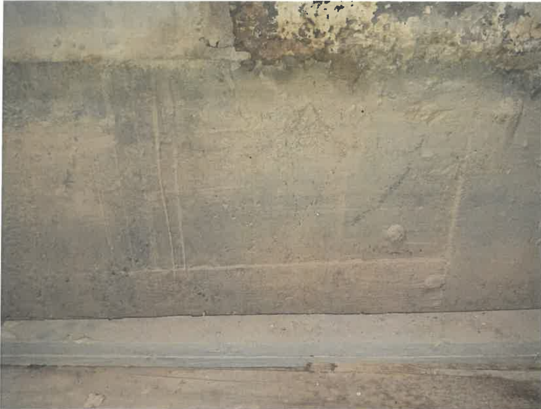
Close-up o the newer concrete at the SW corner
