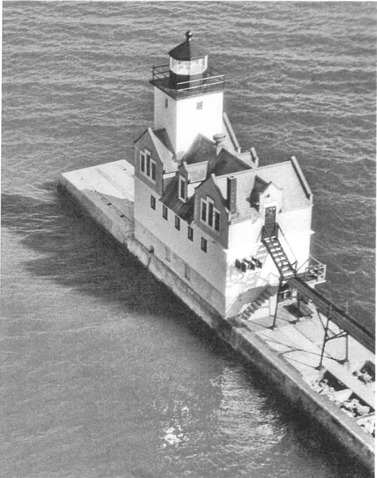
This image (1950s) shows the pier is narrowed and the openings on the original image are already covered over with metal plates, and a small down is under the catwalk.
