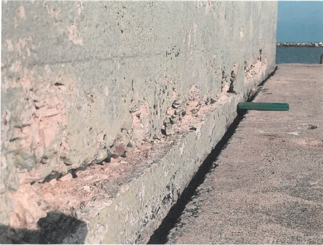
BOTH: East face foundation damage details
