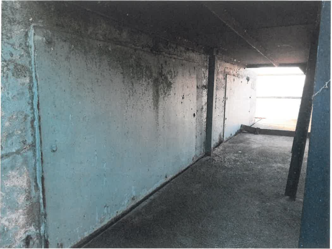
Metal plats on western face under entry deck
