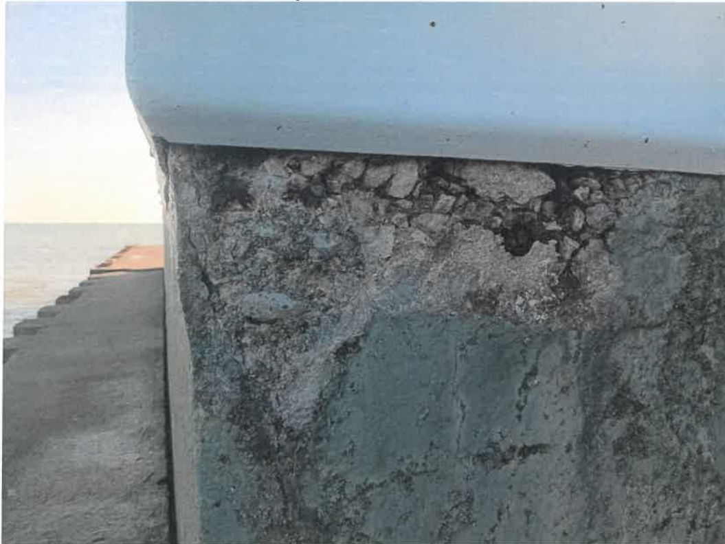
BOTH: KLH detail of concrete damage on NW corner exterior
