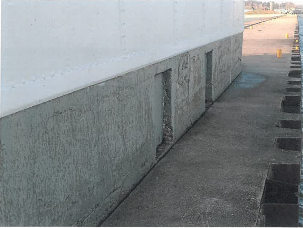
North foundation openings
