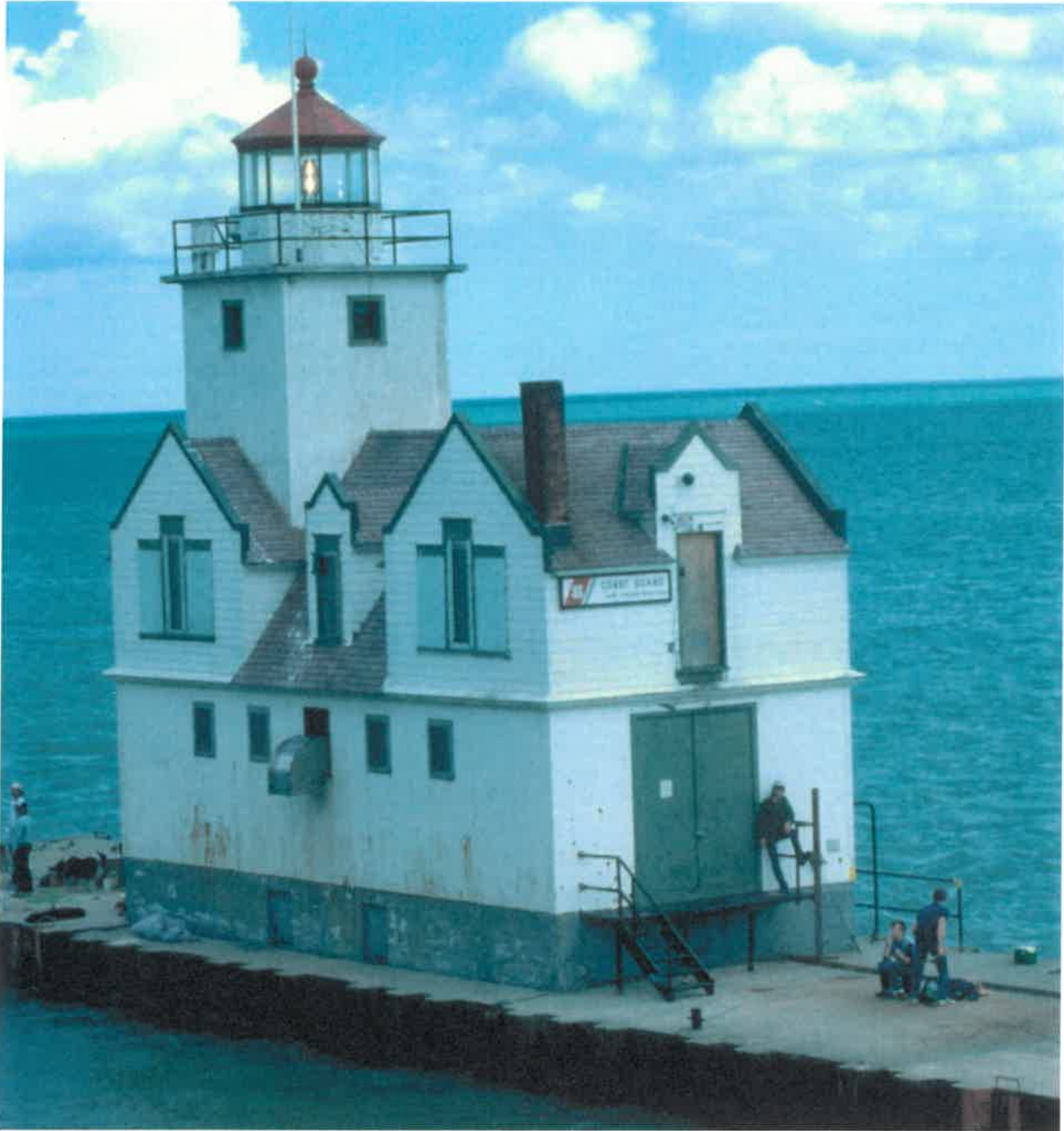
Kewaunee Pierhouse - Shortly after automation – pier is at the same level as the old north openings and there are large metal plates under the deck. ON the right you can see the conduit carrying the 600v power source for the automated system.
