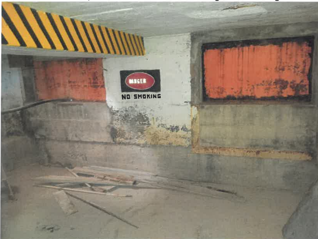
Interior basement looking west.
