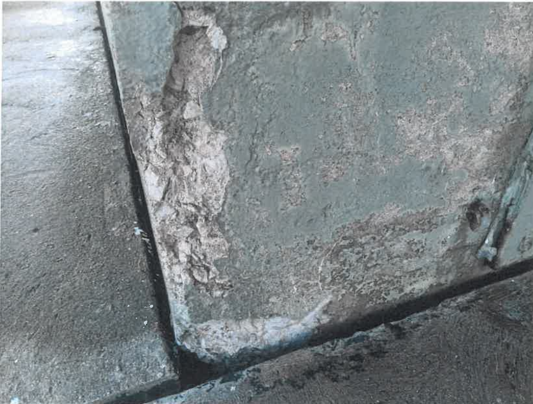
BOTH: KLH detail of concrete damage on NW corner exterior
