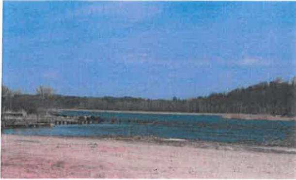
River Landing in progress
